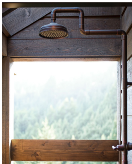
Outdoor shower customized with three 90-degree bends to create necessary height.
