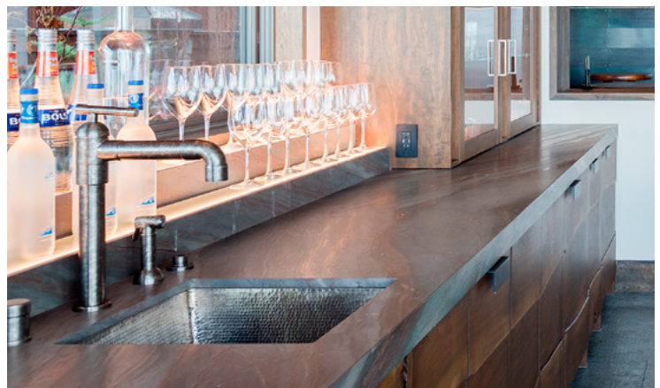
Great room wet bar with Brut kitchen faucet, side spray and air gap in Rustic Nickel
